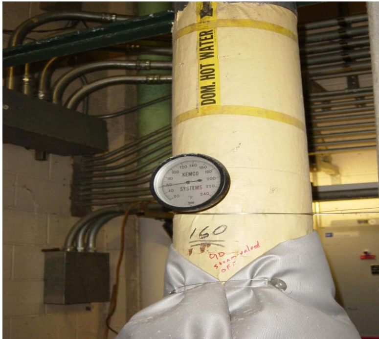
Figure 4. Laundry water feed line temperature gauge, after installation and operation of ozone laundering system.
